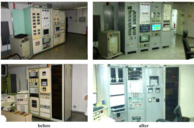
Figure 31. Racks of control and emergency rooms (before and after substitution).
