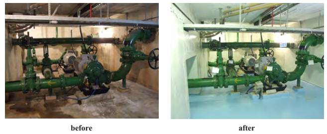
Figure 32. Floor of the engine room (basement floor) and of the reactor hall (third floor) (before and after adequacy).
