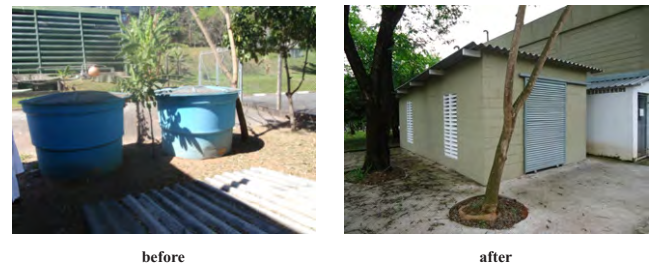
Figure 34. Adequacy of the diesel tank cover.
