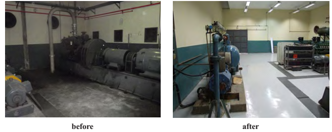
Figure 33. Electrical system building (before and after improvement).
